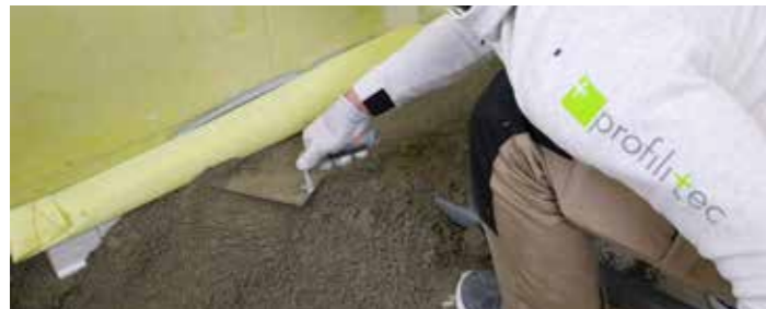
Make the screed by filling also the spaces underneath the channel, until reaching the drain flange.
