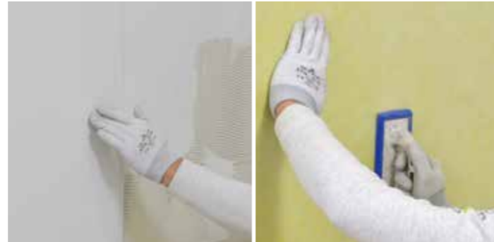
Spread C2-S1 cement-based adhesive, with a notched trowel (5x5 mm), on the relevant walls. Make sure to remove any air bubble that may form during the application of Foiltec using a rubber trowel.
