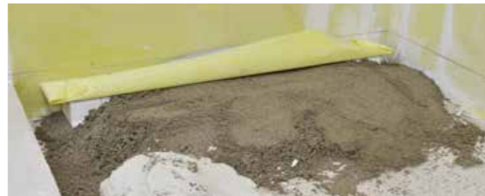
Continue laying the screed with a minimum slope of 1-2% so that the water flows towards the channel.
