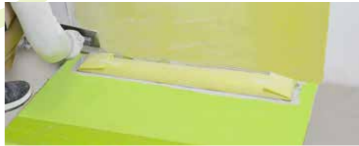
Spread tile adhesive on the surface around the channel by using a 5 x 5 mm notched trowel.
