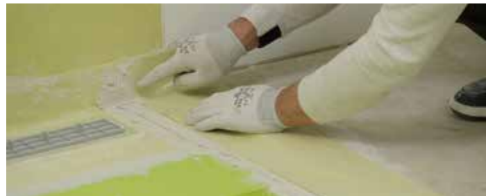
Install the corners and the sealing strip along the junctions between the shower tray and the lateral part between tray and floor.
