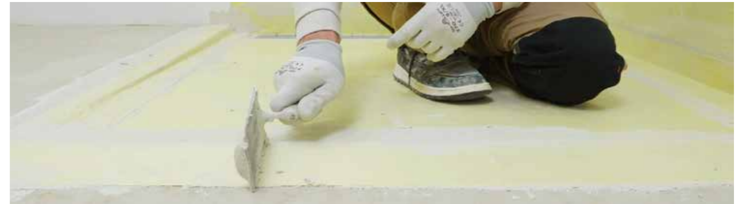
Proceed with waterproofing the entire surface where the screed is present. Before installation, cut the Foiltec membrane to measure.
