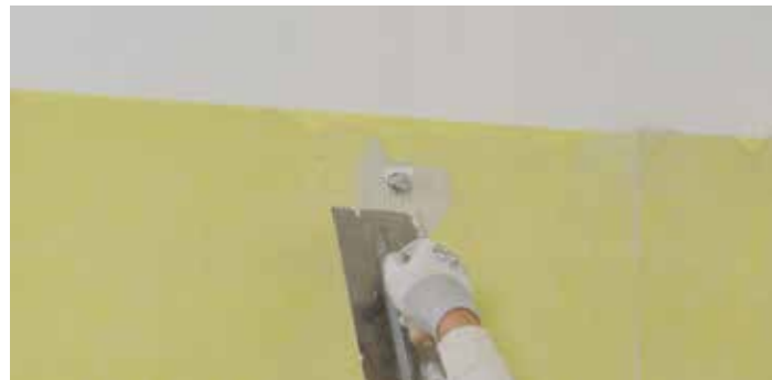
Spread a layer of tile adhesive with a notched trowel around the pipe connections. Then, install the T20 Foiltec junction to waterproof the area around the connections.
