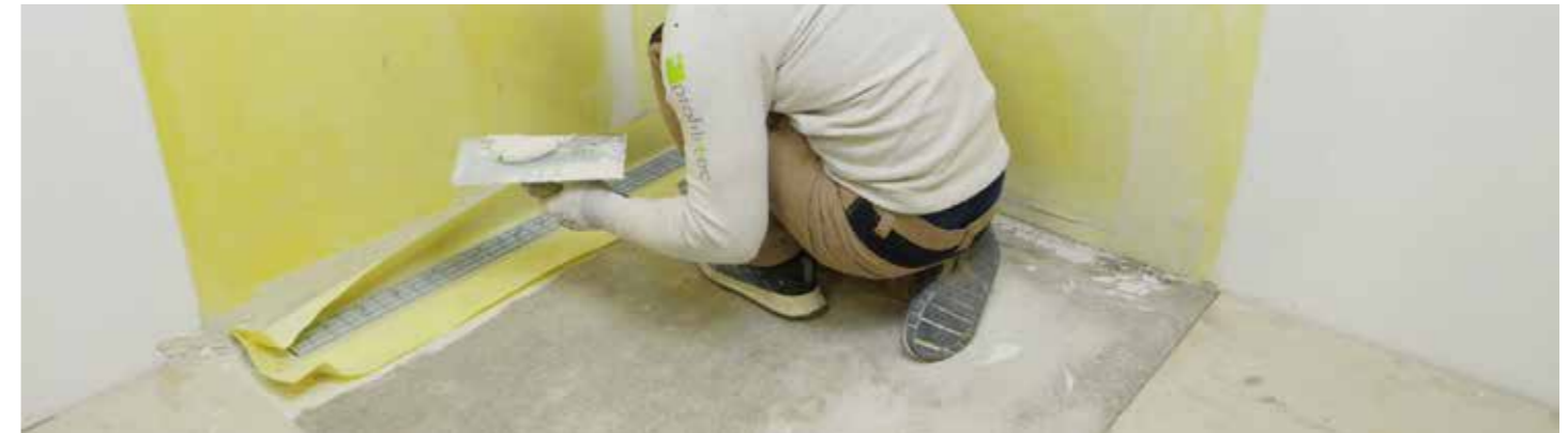
Ensure that the construction plug is properly installed. Spread the pre-attached membrane on the screed.
