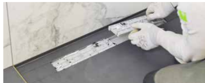
Remove the construction plug.
