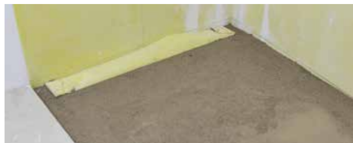
Immediately after laying the screed, make sure that the channel is still in its initial position and has not moved accidentally.
