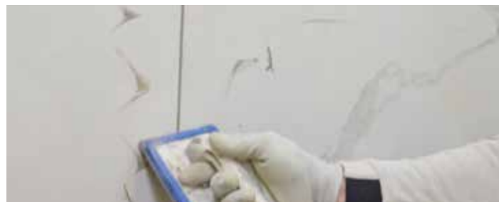
Grout the tile joints.
