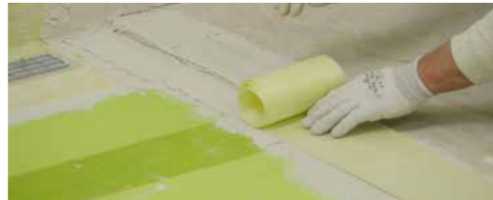
Waterproofing the floor: lay the Foiltec membrane with a notched trowel, approximately 5 x 5 mm. The TRAY tray is already waterproof so you do not need to cover it with membranes.
