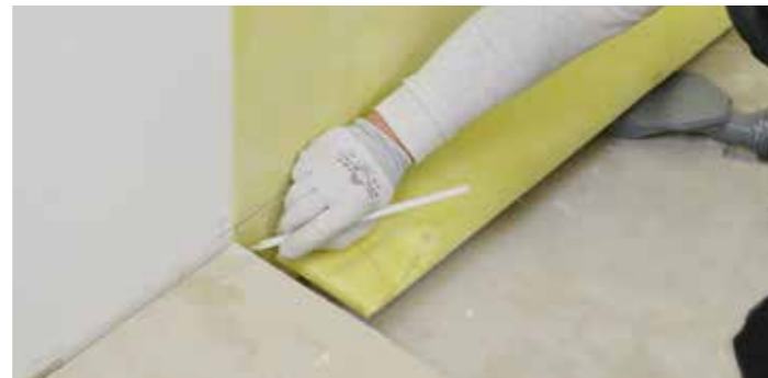
Determine the installation height you want to achieve by considering the height of the channel and the cover, the tile adhesive and the thickness of the flooring.
