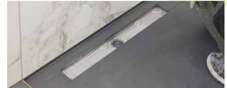
Place the hair trap inside the drain hole.
