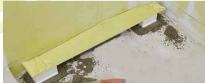
Prepare the piping connection.
