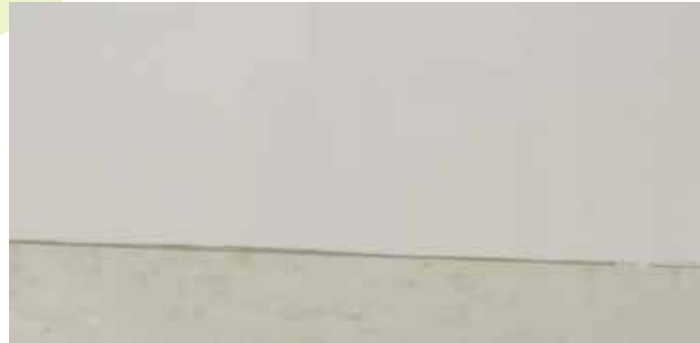
Waterproofing the walls: before doing so make sure they are flat, clean, and smooth.
