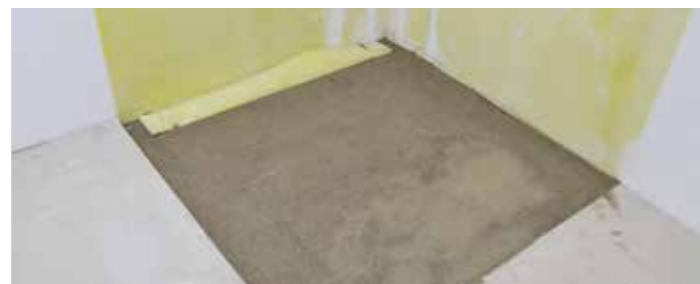
Wait until the screed dries before waterproofing.
