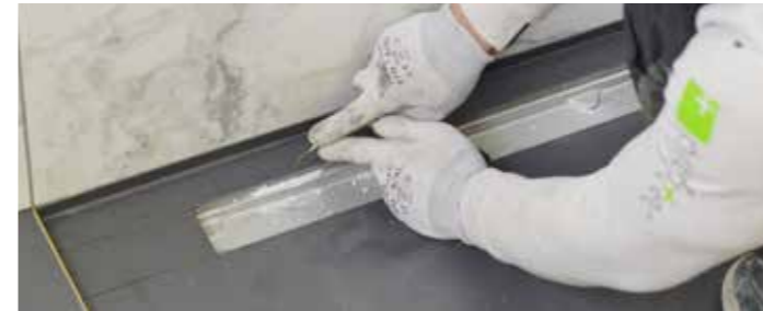
Clean the cavity of the channel from any residual mortar or dust and make sure they do not fall in the drain.
