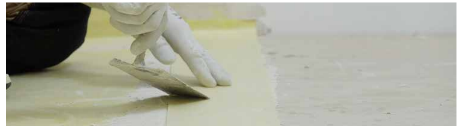
Spread the Foiltec strip on the joints between the screed and the floor.
